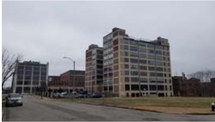
Existing intersection at Locust and 21st Street.
