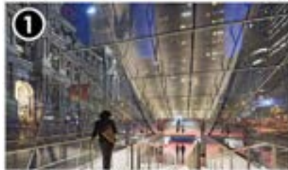
1 Station "daylighting" & enhanced LED lighting
