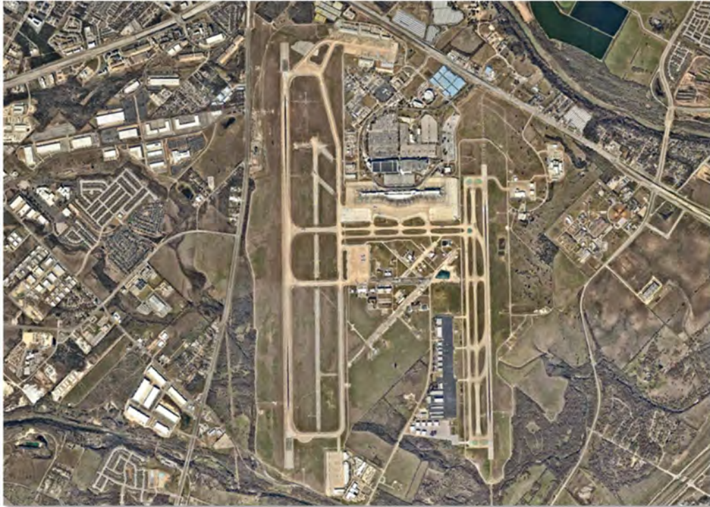
Figure 3-10. Austin-Bergstrom International Airport Aerial
