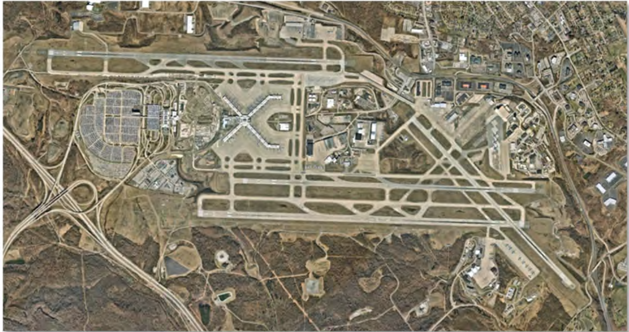
Figure 3-7. Pittsburgh International Airport Aerial
