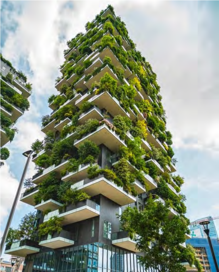
Figure 44 - Vegetation Throughout the Façade
