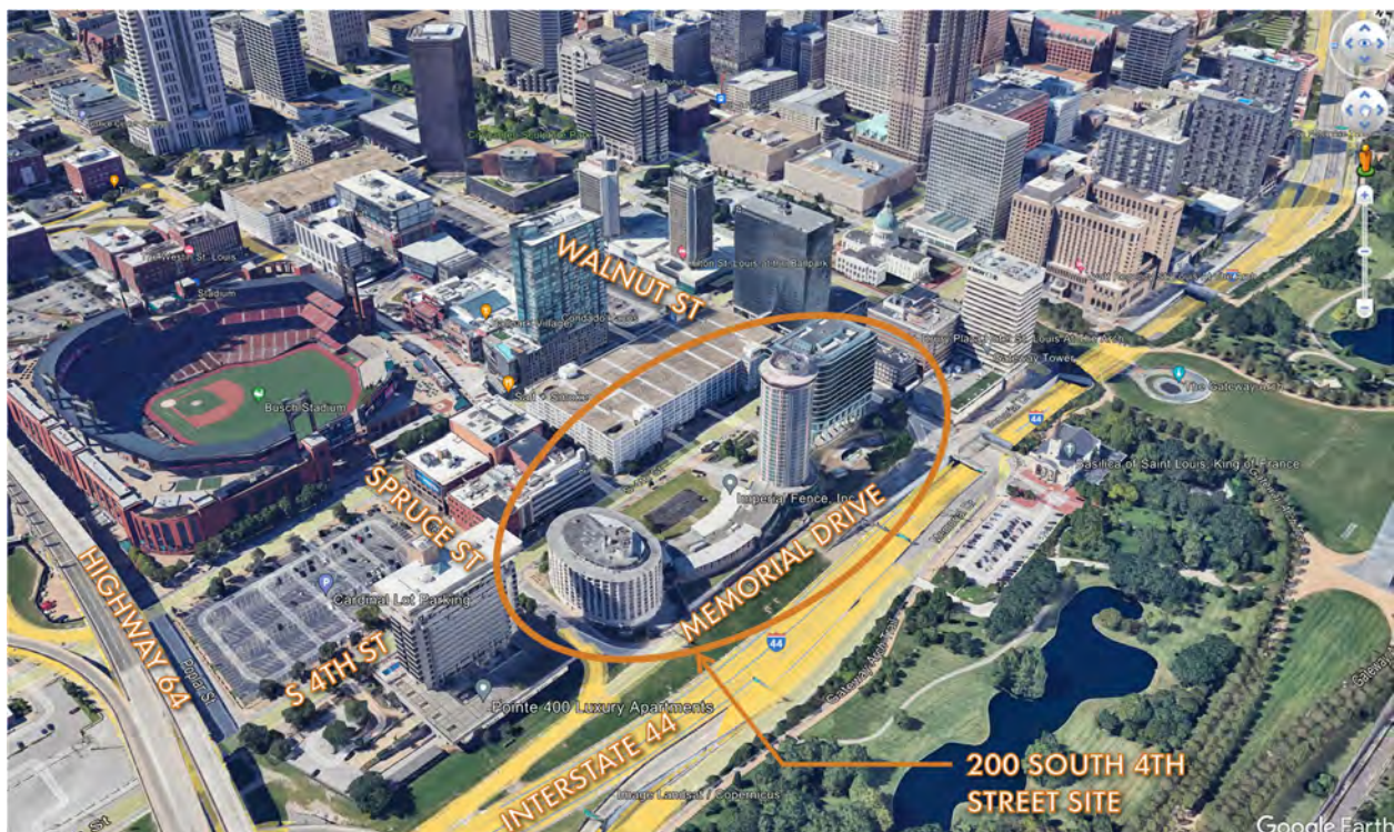
Figure 6 - Aerial Looking Northwest
